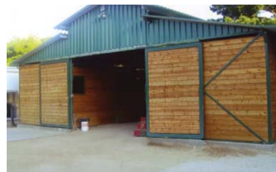
Fully enclosed barn
